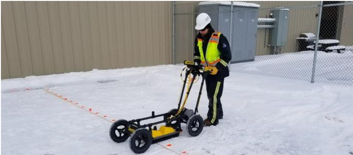
GPR data collection in winter at the Anchorage International Airport
