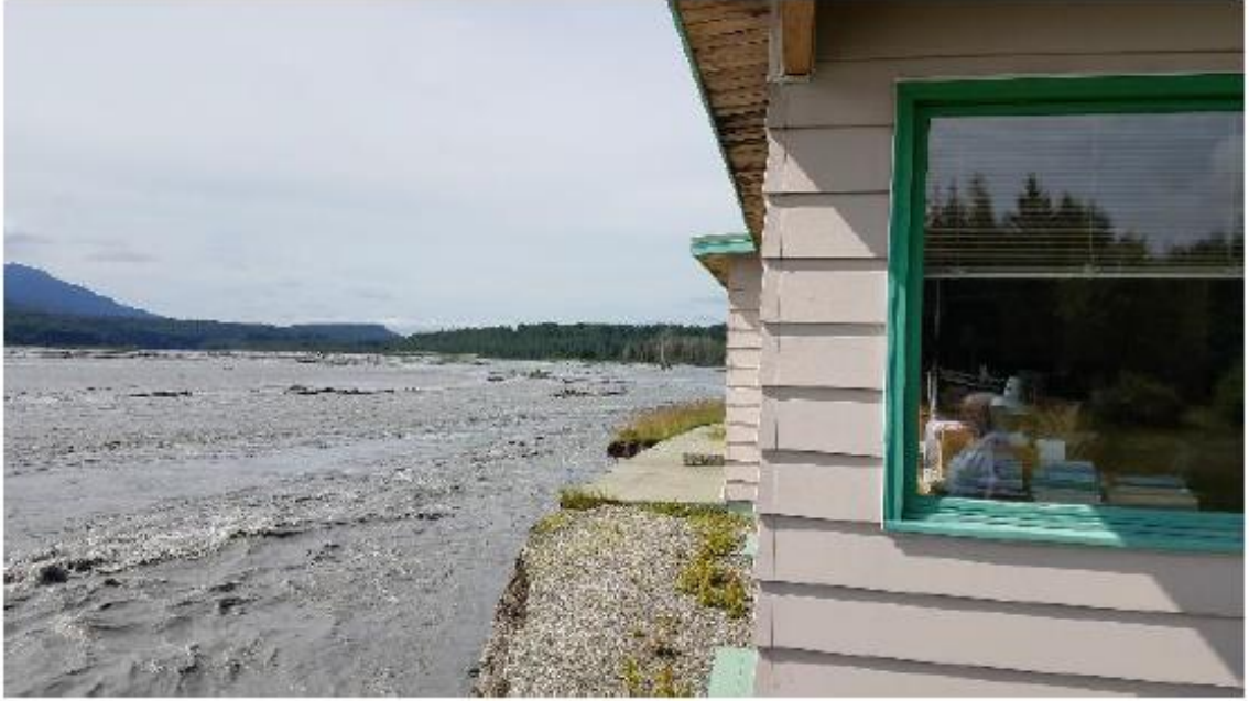
A home on the Matanuska River threatened by erosion. July 7, 2017 (KTUU)
